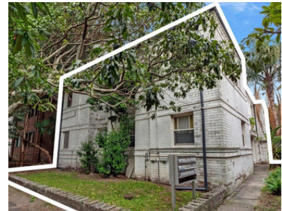
60 Dolphin Street, Coogee
