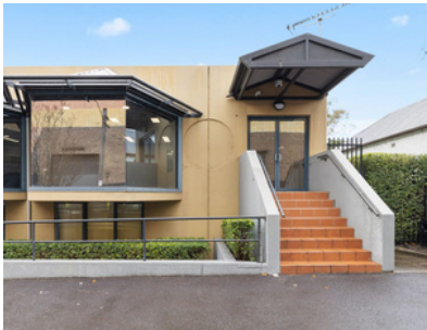
5-13 Parsons Street, Rozelle
