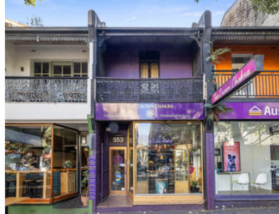
553 Crown Street, Surry Hills
