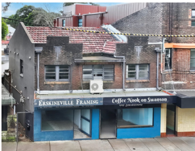
104 & 104A Swanson Street, Erskineville
