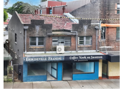
104 & 104A Swanson Street, Erskineville
