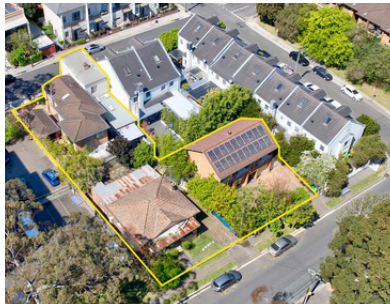
98-100 Wentworth Road & 9-11 Oxford Street, Burwood
